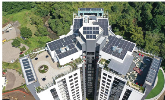
Costa Rica | Apartment Complex
