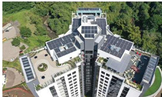
Costa Rica | Apartment Complex
