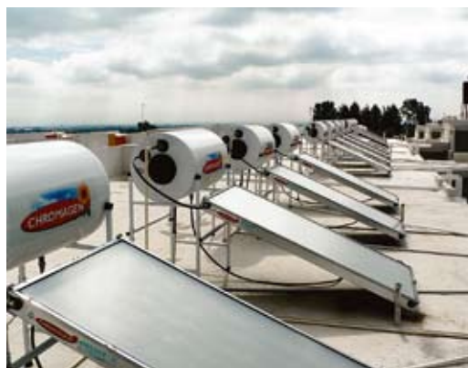
Thermosiphonic systems by Chromagen each with a 150 L tank and one collector.
